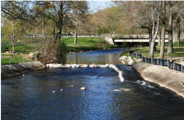
PEQUONNOCK APRON- The water down the sloped concrete apron was too shallow so the team built this sandbag diverter to send all the water to one side where it would be deep enough to allow alewives to swim up. The Bunnells Pond Fishway is about a quarter mile upstream from here, in Bridgeport. (Photo by Gwen MacDonald, Save the Sound)
