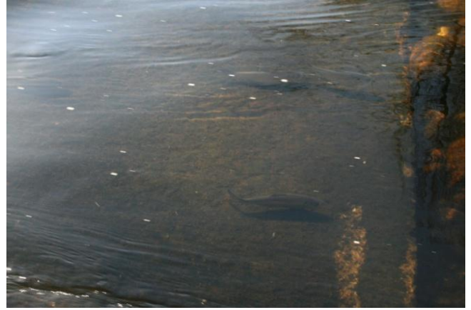
This is the top of the apron where the velocity is the highest. If you enlarge this photo on your screen, you may see one alewife in the middle (casting a shadow) approaching the top and another two or three toward the back also struggling to get up. After the sandbags were placed, this water was about 6 inches deep. A properly designed fishway (ready to be built at this site this coming summer) will manage the flows properly to keep them at suitable depths and velocities that will allow alewives to pass easily. (Photo by Gwen MacDonald, Save the Sound)
